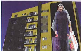
The DMU Cube, which opens in Leicester this month, will house not only the city's new Phoenix arts cinema, but also an innovative digital art space. The building, on Leicester's Phoenix Square, contains 63 new homes, seven office studios, 22 managed workspace units as well as the cinema and gallery, which will also feature exterior exhibitions like Martin Rieser's Songlines , pictured.
